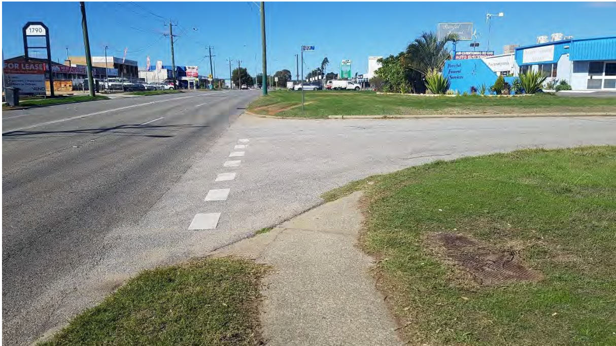
Photo 11: Narrow footpath with non-standard pedestrian ramp. Footpath does not continue on far side of Ozich Court.
