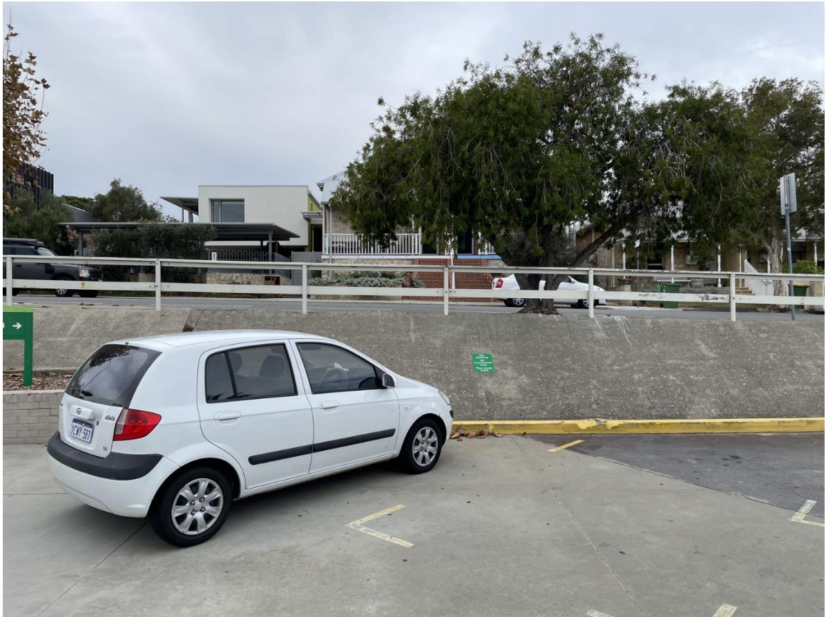
Elevation at rear of subject site
