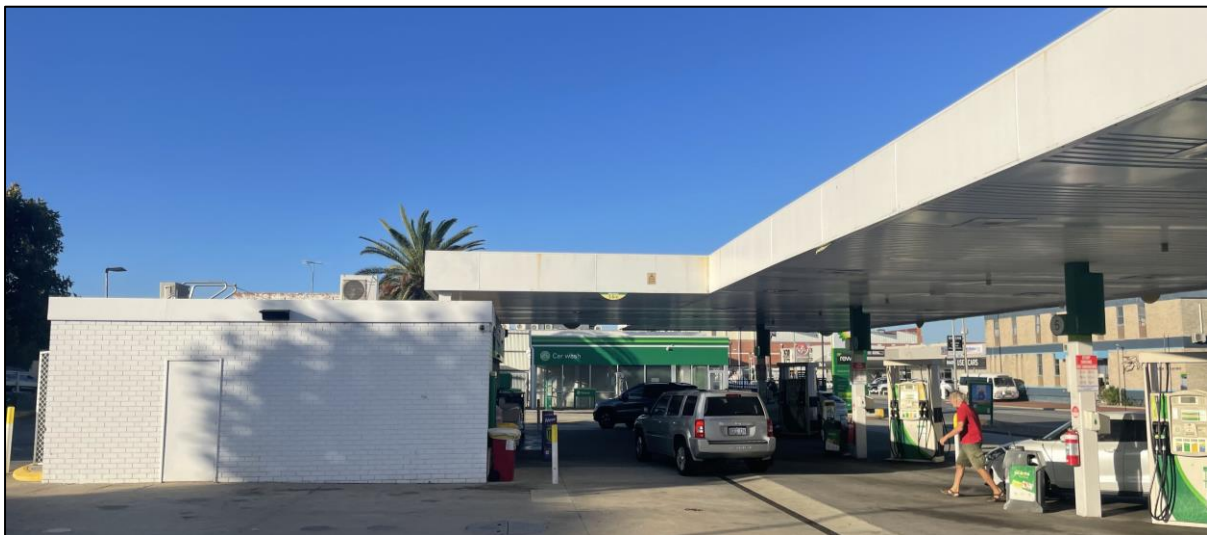
Photograph 5 – Northern façade and canopy, looking south.
