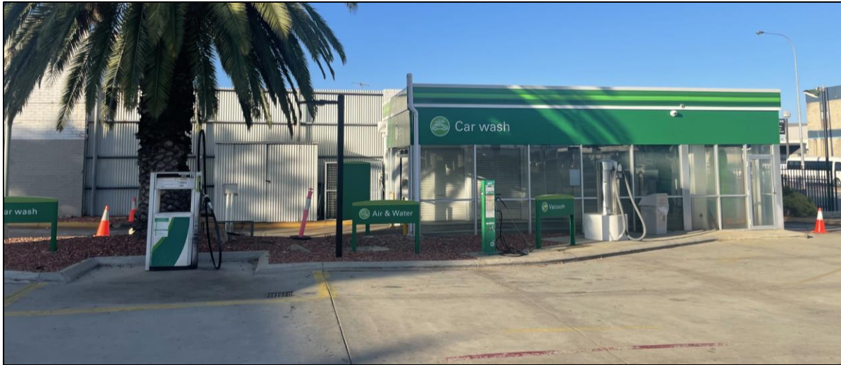
Photograph 4 – Existing drive-through car wash, diesel bowser and air/water bay on the southern portion of the site, looking south.
