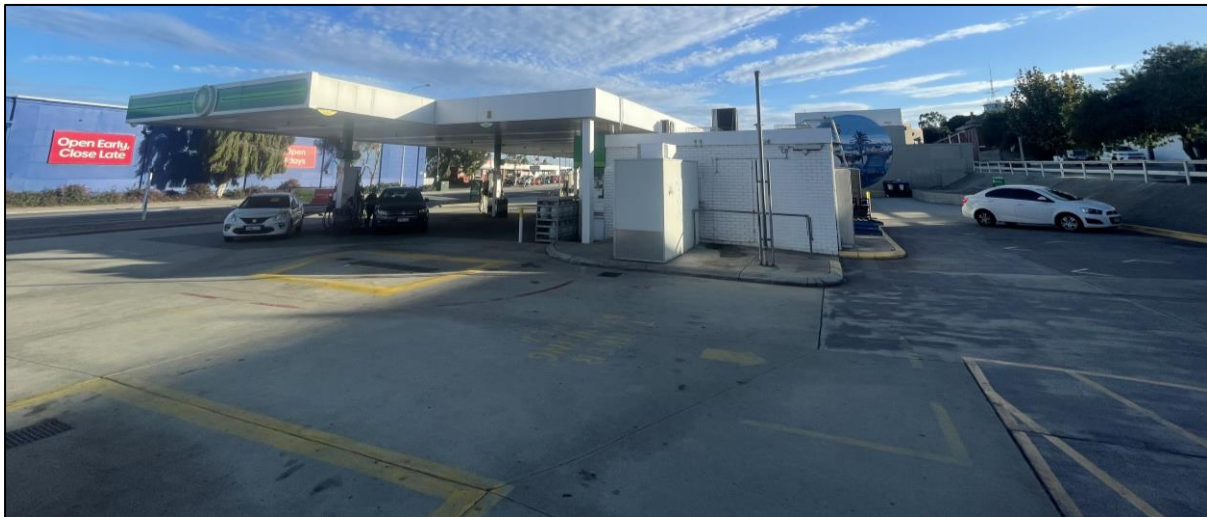
Photograph 2 – Subject site from the south eastern portion of the site, looking north west.
