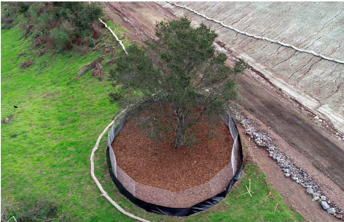
Figure 2 TPZ installation with mulch coverage
