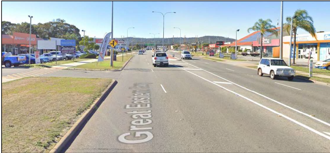
Figure 4. Eastbound view along Great Eastern Highway
